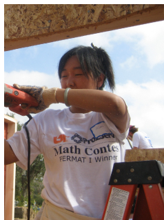
(BELOW) Eileen Zhao, TN A, saws wall openings.
