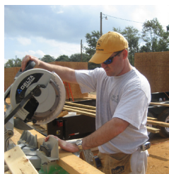
Harold Z. Eubanks, AL E, cuts lumber for more framing work.
