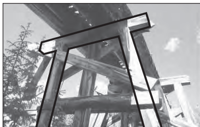
Above: The bent on a trestle bridge is key to giving the structure its integrity.
