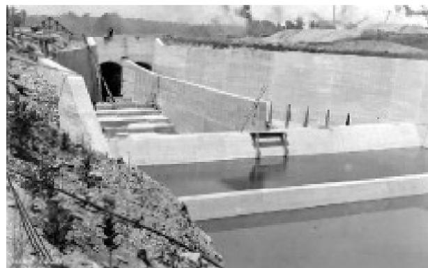
removed just before water was allowed to enter. The finished permanently open outlet conduit at Englewood Dam is shown on June 28, 1919 (right), just before water was allowed to enter. View is looking upstream from the end wall at the base of the spillway toward the dam, showing the stair-step structures on the spillway's floor (water would flow toward the viewer and off to the lower right).
